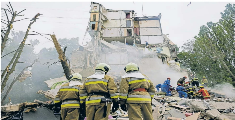
DESPERATE SEARCH: A Russian missile-and-drone barrage Thursday on Kyiv destroyed an apartment building and left 13 people dead, including a 6-year-old boy. It left the highest number of children injured by a single attack in the war. A7
